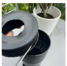
Trim the lower flange with a good pair of kitchen scissors. (Shown here for fitting to round downpipe)
