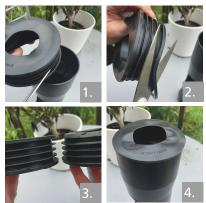
Trim the lower flange (only) with a good pair of kitchen scissors. (Shown here for fitting to round downpipe). Note 3rd photo shows before and after with grommets held upside down
