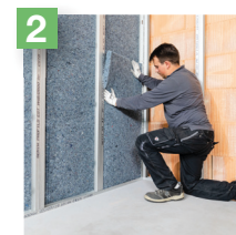
Laying the second layer of insulation
