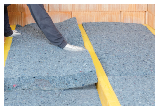
Double layered in cross layers is possible
