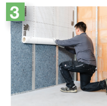
Installation of the vapour barrier
