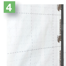
Fixing the vapour barrier with double-sided adhesive, creates a technical vacuum then install the facing plates
