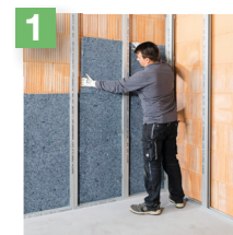
Laying the first layer of insulation
